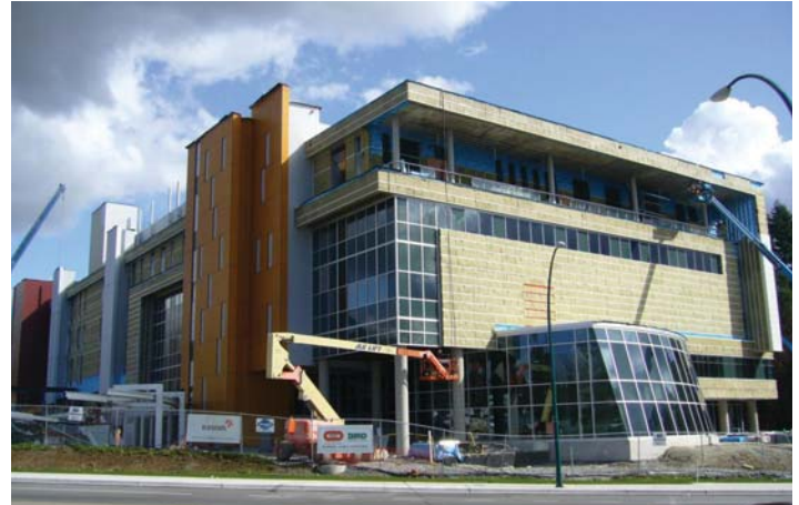
Construction of Surrey Outpatient Care and Surgery Centre
